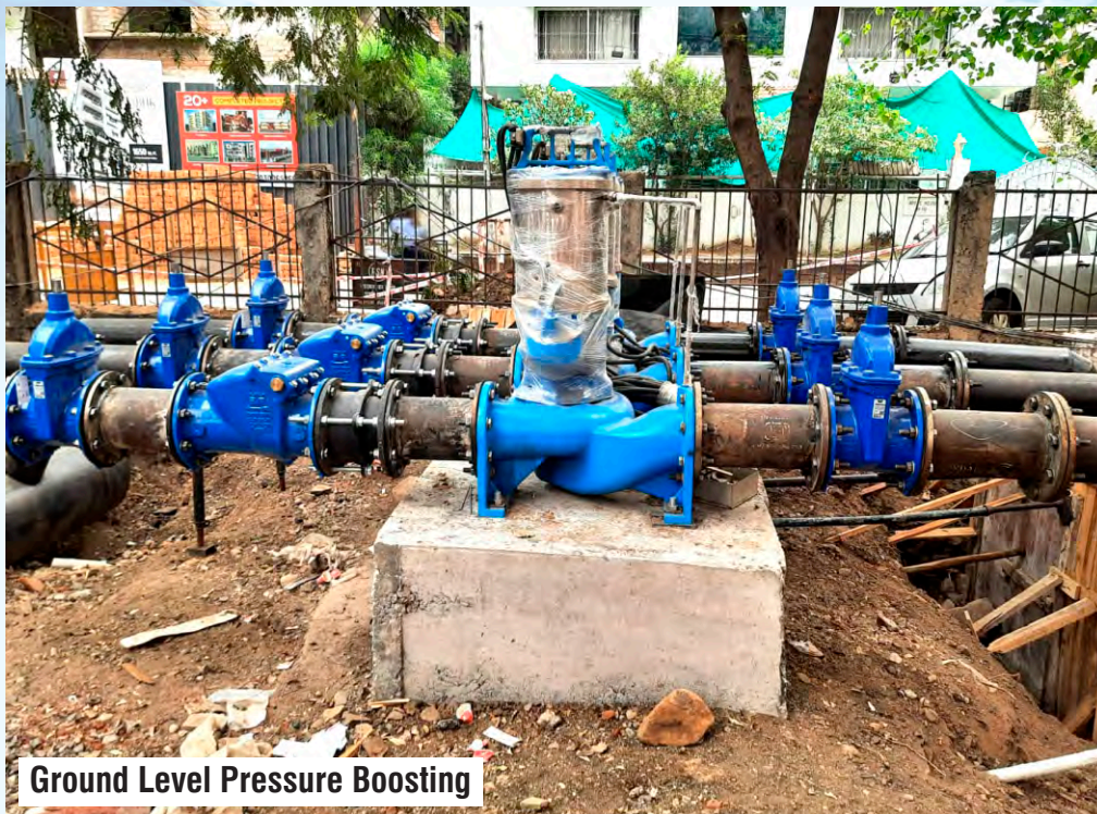
Below Ground at Main Pipe Level ....& the Surrounding Pit can be constructed later on....
