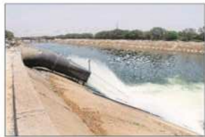
Water from the Mahi river being lifted and drained into Narmada canal that supplies drinking water to two-thirds of Gujarati population. Jitendra Raju
